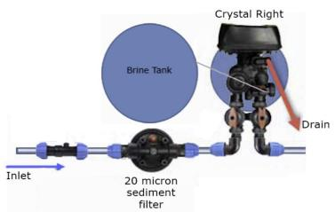
In this example a 20 micron sediment pre-filter has been added. The crystal right system is fitted with a bypass valve so that the system can easily be isolated and the inlet water will bypass the system so there is no loss of water.
